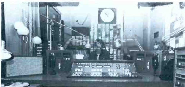
Figure 4 The WPLJ main air studio (FM-1), as seen from the engineer's side, is similar to that of 8A, but faders 8-10 are used for turntables.
